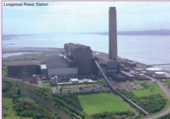
Longannet Power Station
